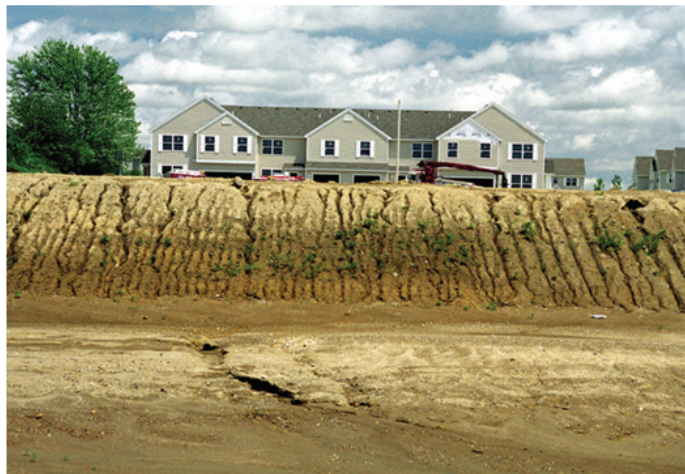
Construction sites can be the source of eroded material.
