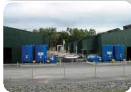
Compressor station in Pennsylvania. Photo by Margaret Brittingham/Penn State Marcellus Electronic Field Guide.
