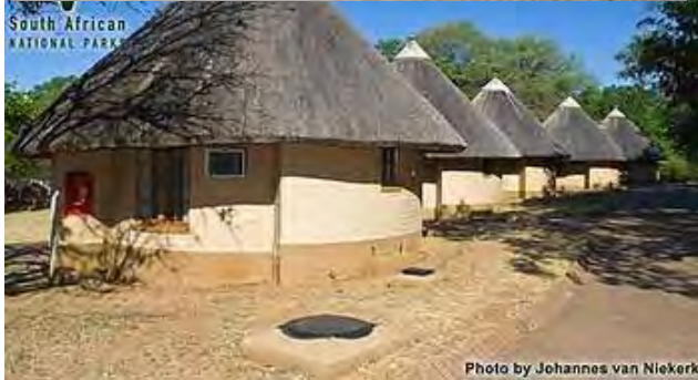
Figure 3: Typical hutted accommodation, Skukuza rest camp
